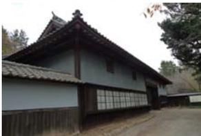
"Negishi-family's terrace house gate (Negishike-Nagayamon)" where is the city specification cultural property building completed the repairer works in November, and faced the completion ceremony in December. The purpose of this repair was to restore the distorted roof, and to have prevented the leak in the roof.
